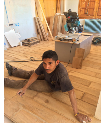
Installation of American oak parquet on the Costa Brava, Catalonia, Spain, 2016
